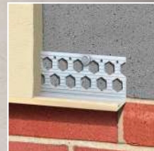
Bellcast / drip beads
